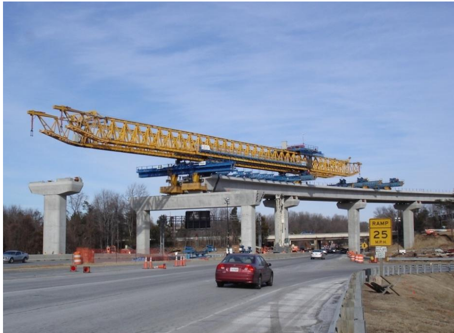
Figure 3. Example of Self-Propelled Bridge Transport. Installation of bridge elements along the corridor of the Washington DC Metrorail Extension Project.
