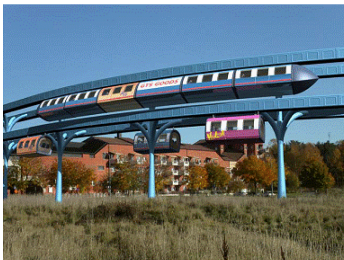
Figure 3.2. Train formation at high speed and separated vehicles at low speed. Picture: Visulogic. Copyright: SIKa
